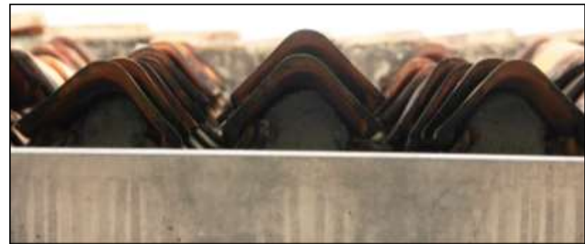
Plate 7.39: Layered Indian 'V' shaped terracotta tiles for roof covering.
