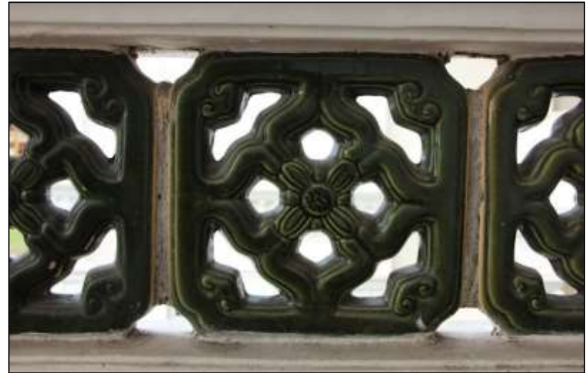
Plate 6.71: Chinese ventilation block outside the room.
