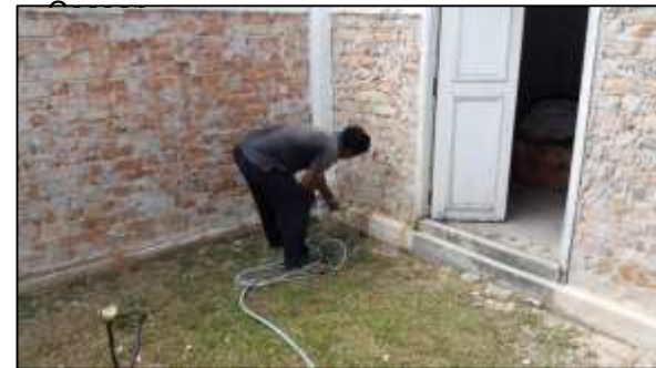
Plate 7.50: Pressure injection process done by
