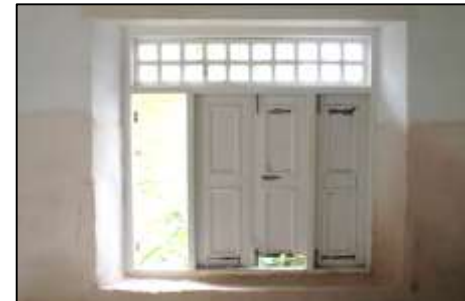
Plate 7.47: Damaged windows with a missing piece.
