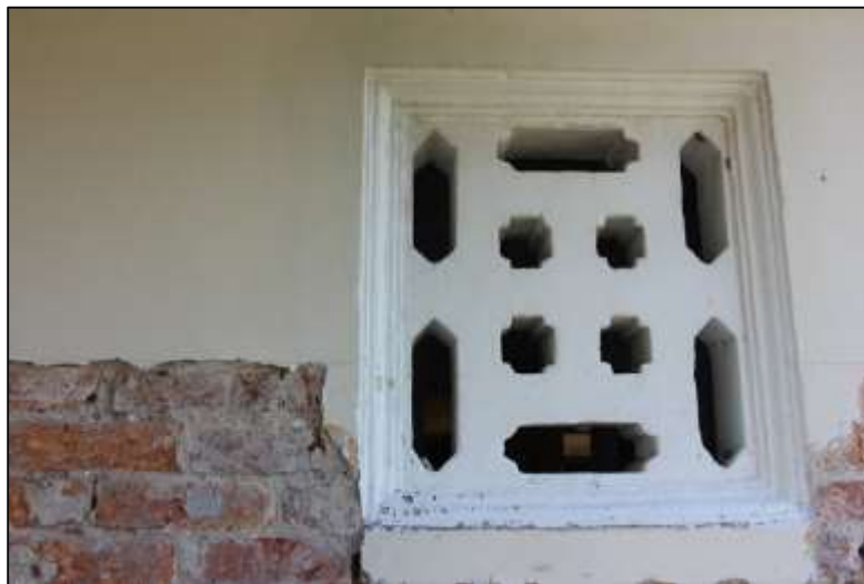
Plate 6.72: Chinese Ventilation Block at Veranda.
