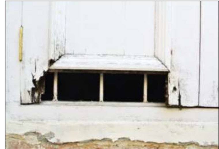
Plate 7.17: Corroded timber window.
