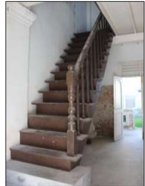
Plate 6.56: Double dog leg staircase at the front entrance.
