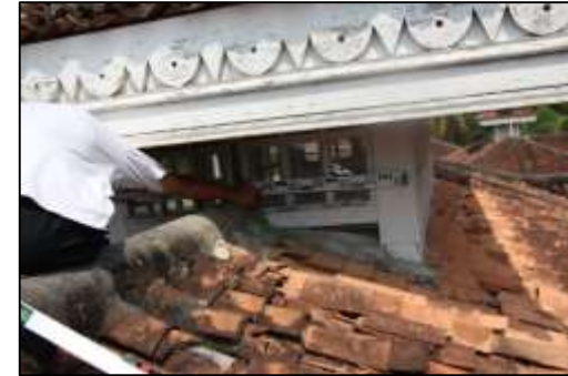
Plate 7.52: Broken roof tiles near the roof lantern.
