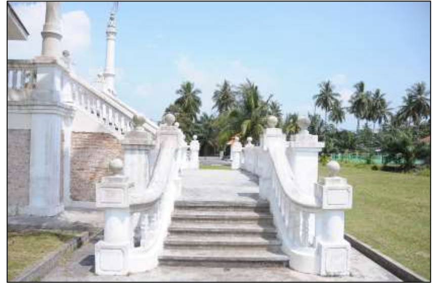
Plate 6.56: Double dog leg staircase at the front entrance.
