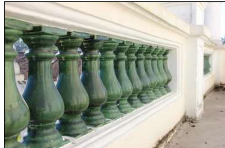
Plate 7.20: Baluster made of porcelain located at the balcony at the first floor.
