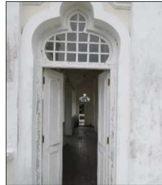
Plate 7.14: The use of glass at the door with pointed trefoil arch.
