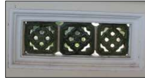
Plate 4.2: Chinese Ventilation Block.
