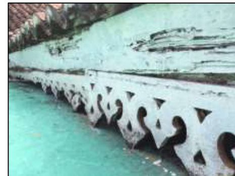
Plate 7.48: Deterioration of wooden ornamentation.
