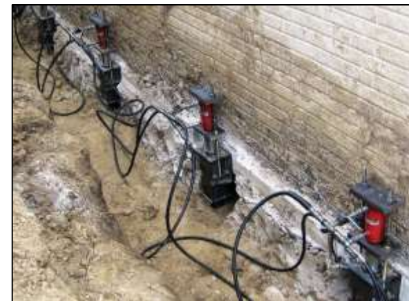
Plate 7.43: Hydraulic jacking.
