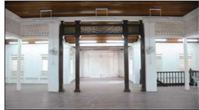
Plate 7.1: Column, Ceiling, Floor Decking Made Of Cengal Timber.
