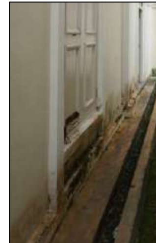
Plate 7.25: The exposed lower part of the building shows the strip foundation of the palace.
