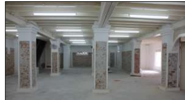
Plate 3.19: Stripped off Columns.
