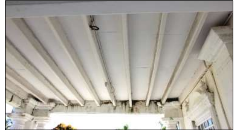
Plate 7.31: Exposed floor girder can be seen at ceiling of the porch and the assembly hall which showed the exposed beam structure of the Istana .
