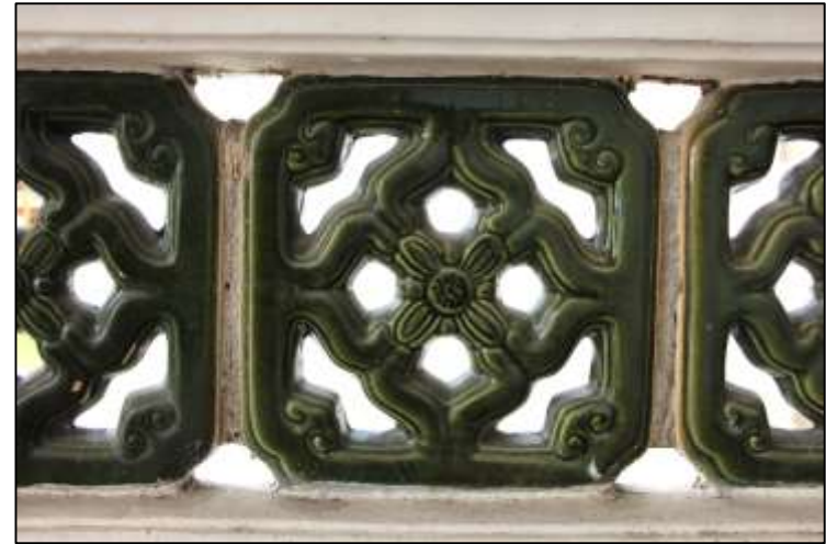
Plate 7.19: Chinese ventilation block made of porcelain.
